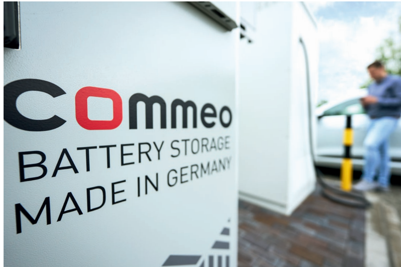
Dream team: The charging infrastructure consists of an electric charging column and a battery system in an outdoor enclosure from Rittal (at the rear).
